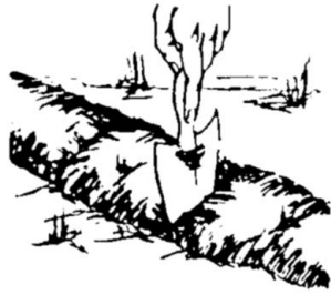
Make an excavation across the tunnel.
